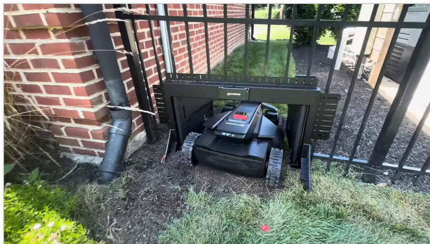
Figure 6. Method B: cut each picket at the top of the gate outline and remove only the lower portion. The picket ends left above the cut become the bolt points for the gate's top rail; the outer pickets take the side bolts.
